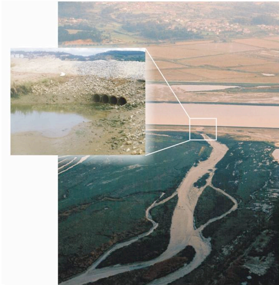
Figure 15. The communication between the two arms of the Mondego estuary after the Northern arm interventions in 1994. Detail of the water pipes.
