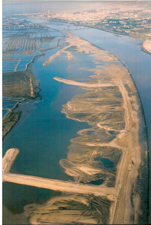
Figure 14. Final interventions at the North arm of the Mondego estuary. Situation in 1994: area between the commercial harbour (at the mouth) and the point of separation of the two arms. Detail of the left margin's land filling process.
